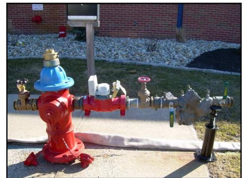
Example of a Hydrant Meter Assembly
